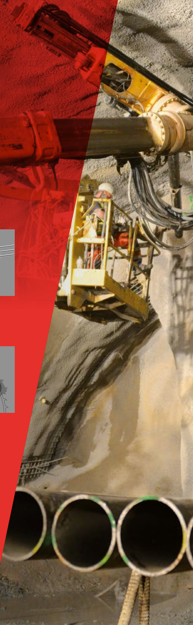
Single AT – Pipe Umbrella with Double Overlap
